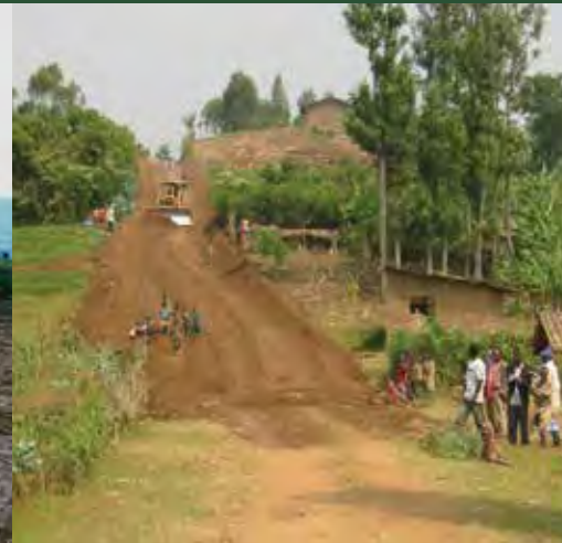
Building the 4 km road
