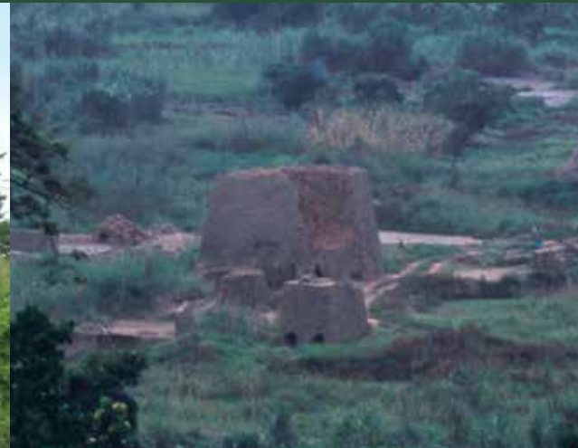
Illegal brickworks in wetland near lodge
