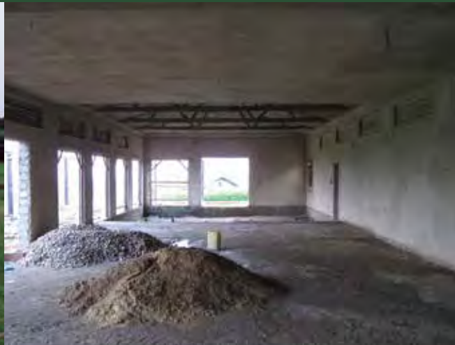
Renovating the old coffee shed
