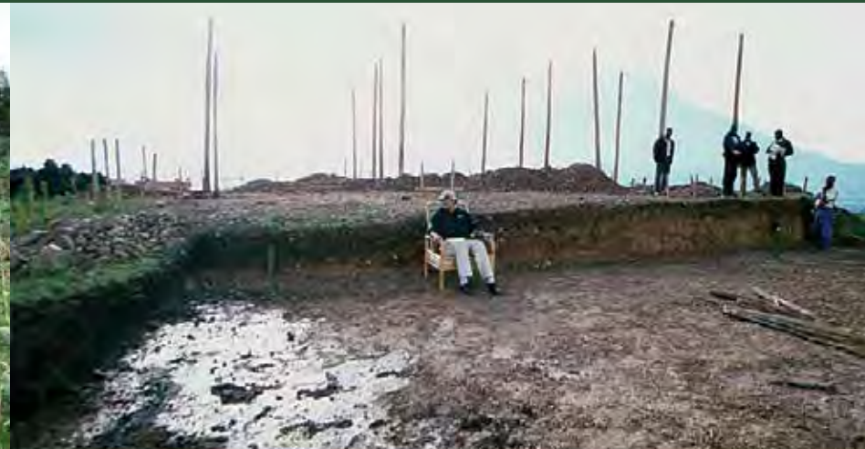
Praveen overseeing foundation work
