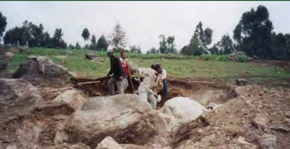
Preparing the site
