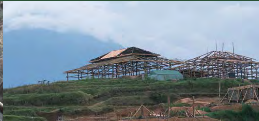
Building the public areas
