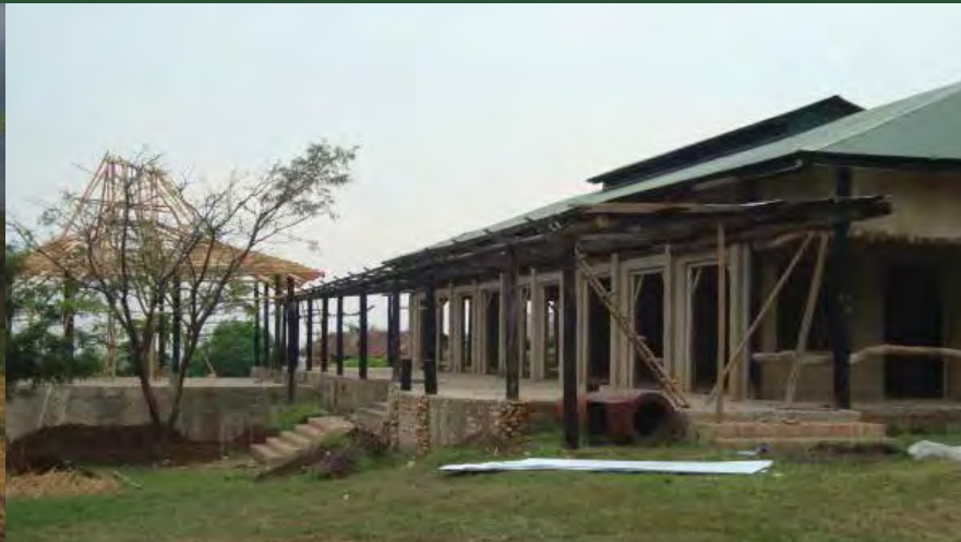
Main building remodelling
