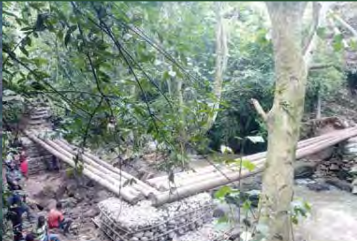
Building bridge across river
